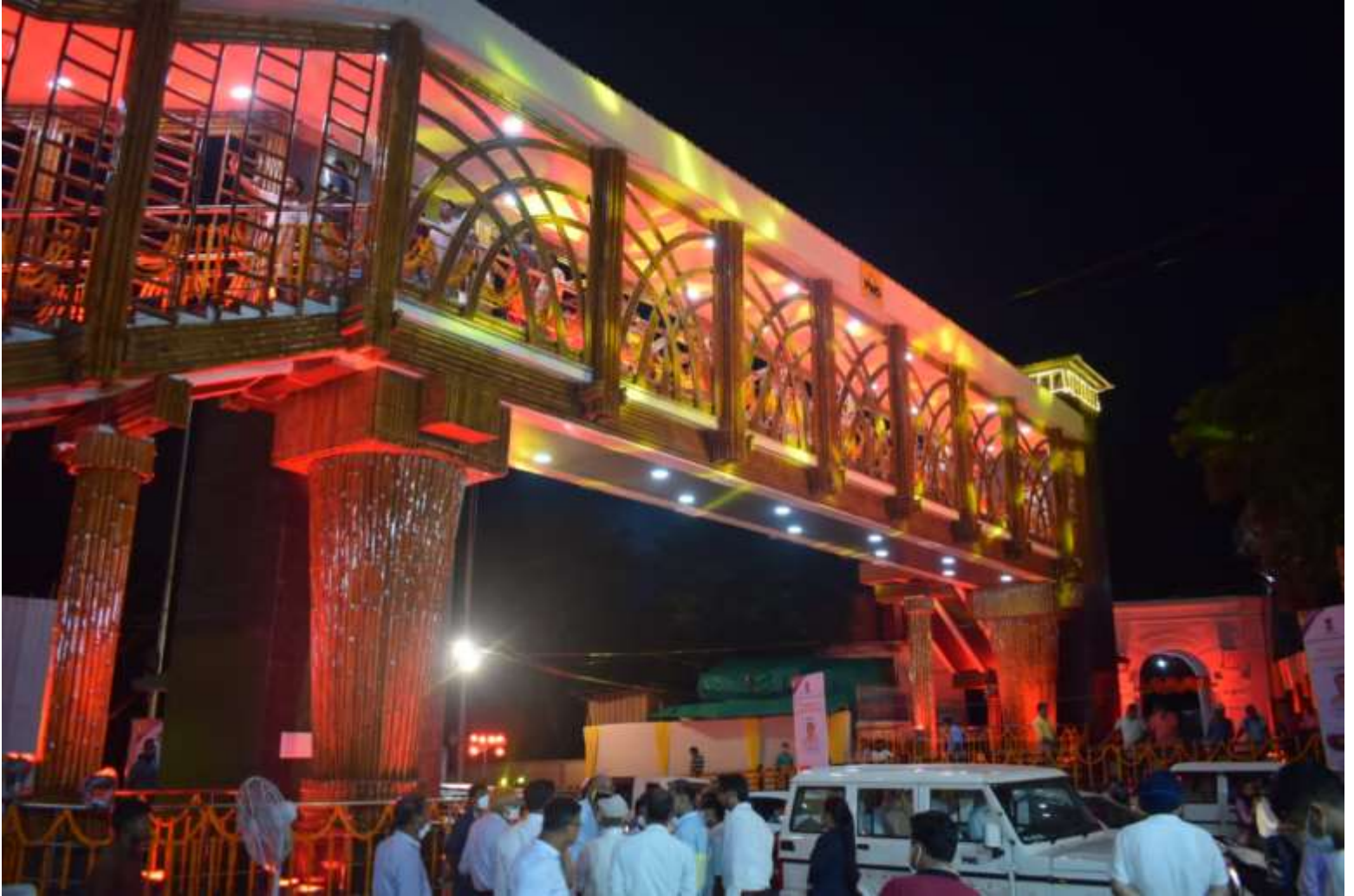
Flyover made of bamboo at Guwahati
